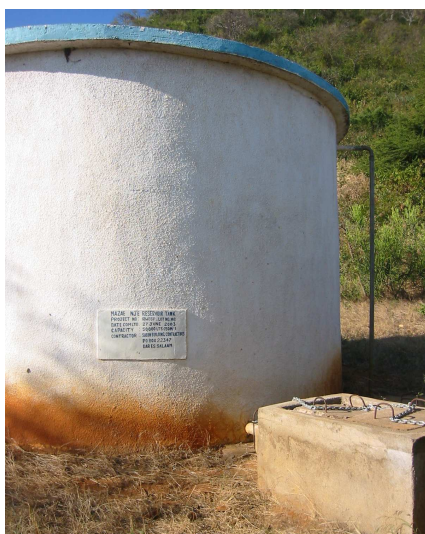
Figure 4.4. Storage Water Tank (gravity system) in Mazae Nje (Mpwapwa).
