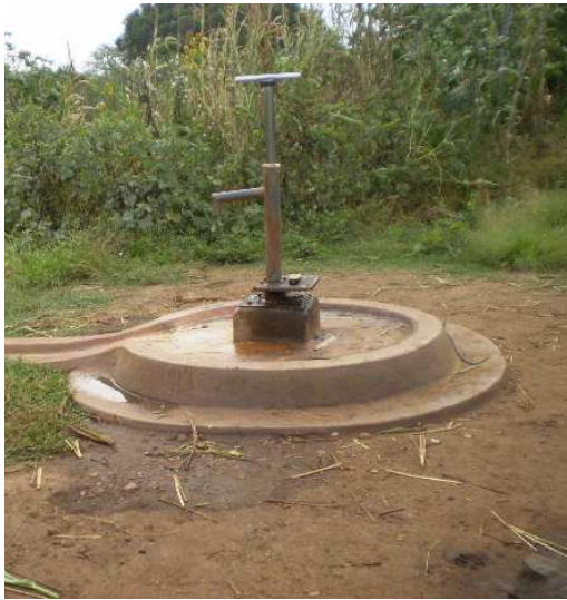
Figure 1.6. Handpump in a shallow well (WA, in Isinghu - Mpwapwa).
