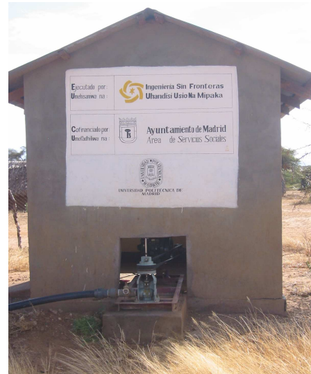
Figure 1.7. Diesel Engine to pump water from a deep borehole to a gravity system (ISF, Mang'ola - Karatu).
