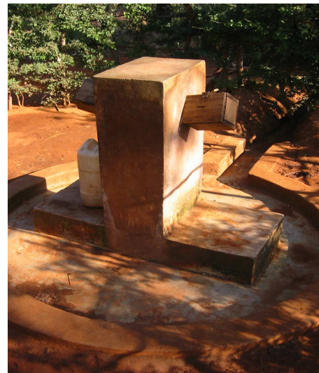
Figure 1.9. Multiple Waterpoint in a gravity system (WB, in Mazae Nje - Mpwapwa).
