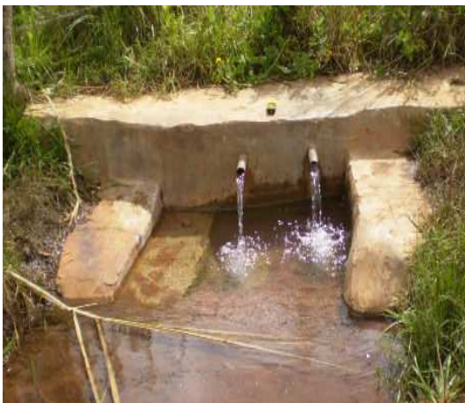
Figure 3.6. Spring protection in Lwihomelo (Mpwapwa).
