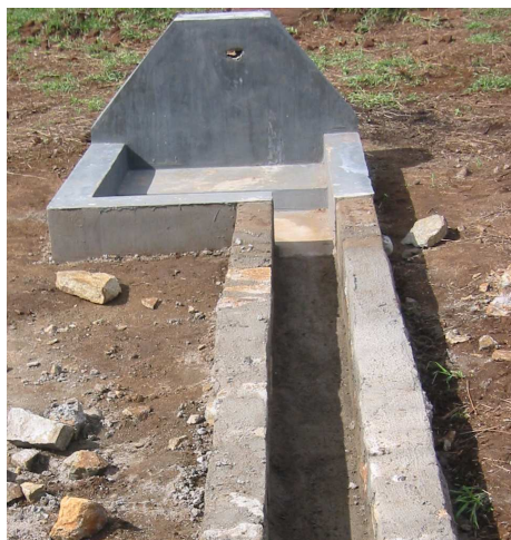
Figure 5.10. Construction of a communal waterpoint (Njoro, Same)
